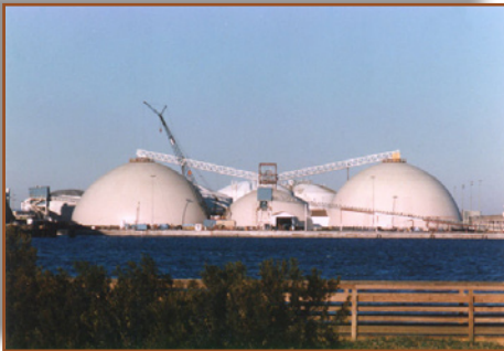
Monolithic Domes as bulk storage for phosphates.
