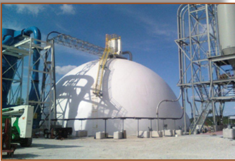
Limestone storage dome
